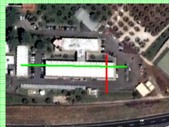
Fig 2. Esrin Building 14 – Aerial view – Radar – Optical Image
